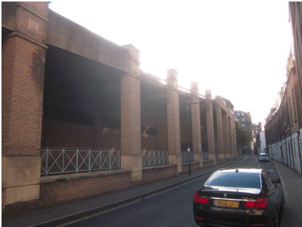
Pre-demolition Photos of Rear (top) and North Elevations in Redan Place (bottom).
