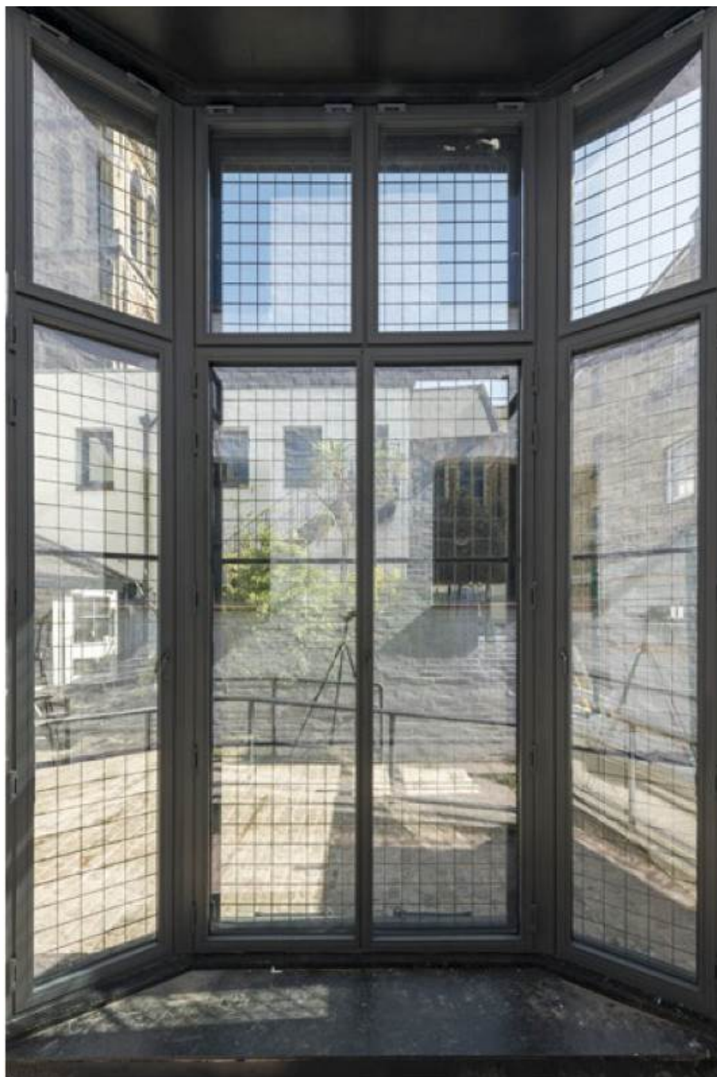
Internal Photo of Full Size Window Mock-up
