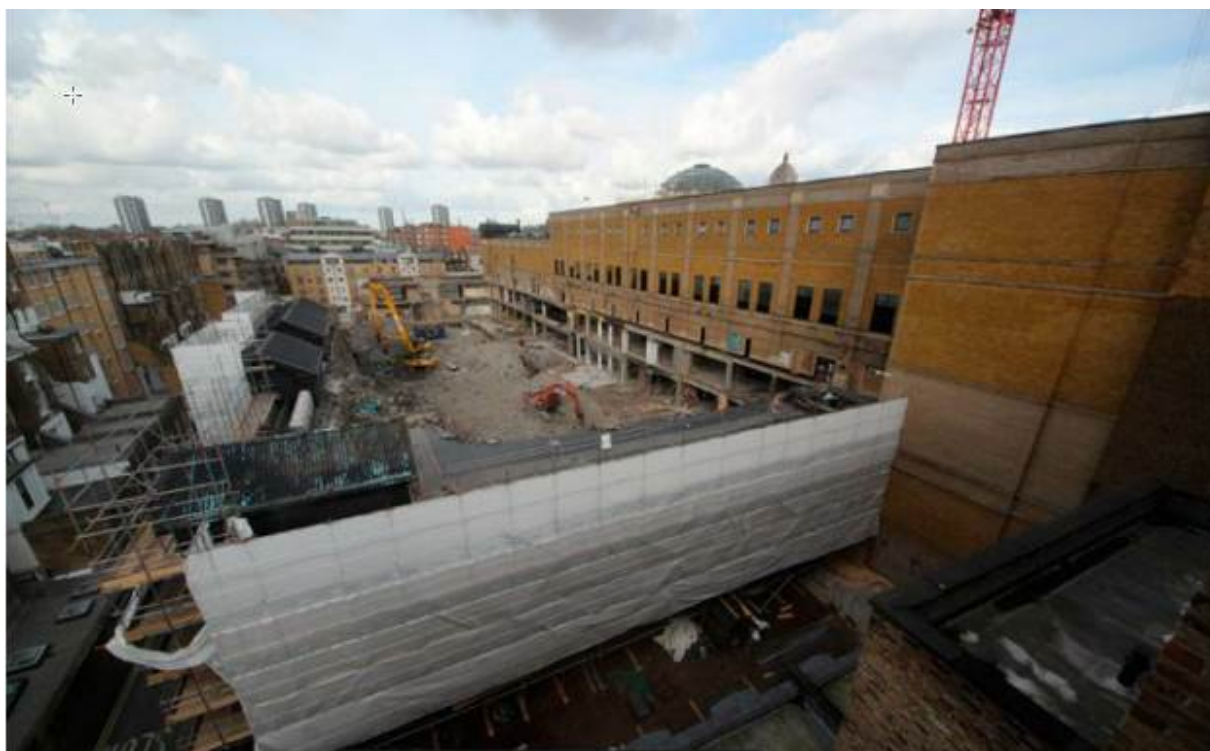
Demolition Works On-site (March 2019)
