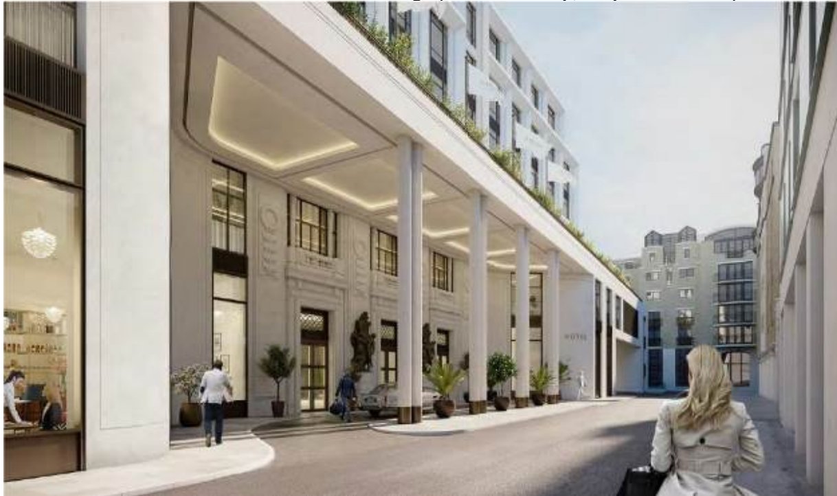
Image showing proposed hotel entrance (left of image) servicing bay entrance (right).
