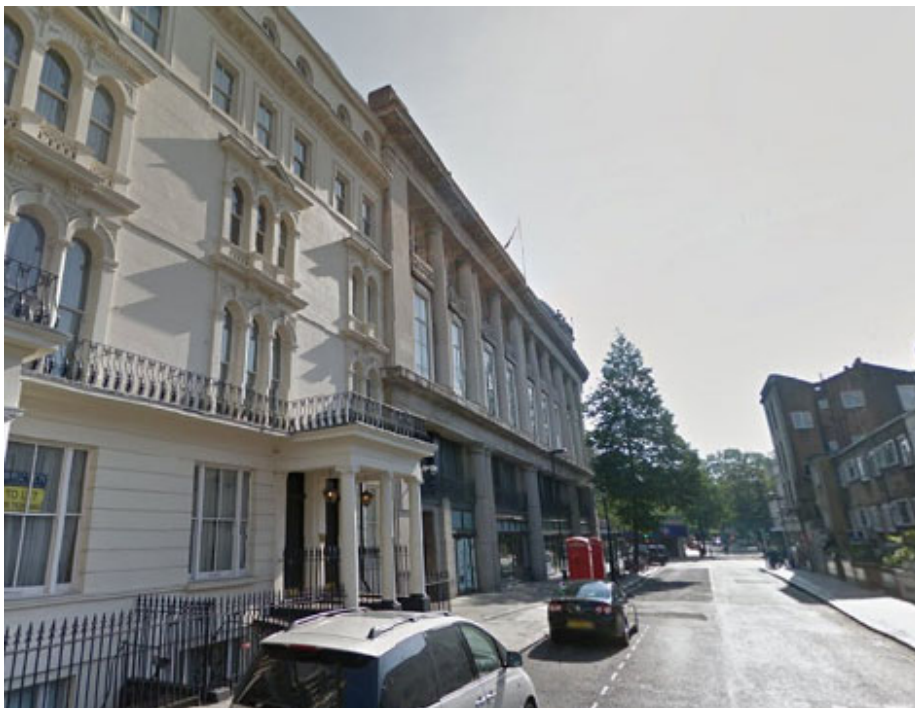
Pre-demolition Photos of the Front (west) elevation at corner of Queensway (top) and Porchester Gardens (bottom).
